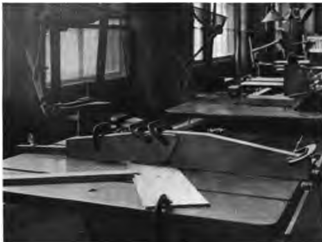
Fig. 3. Saw-Guard for Special Work. (Eastman Kodak Company.)
